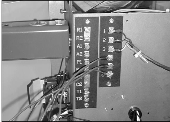
Connections for BMS control are made to the terminal strip located on rear of PRIMERA control box. The terminal strip is accessed by removing the PRIMERA top pan.
